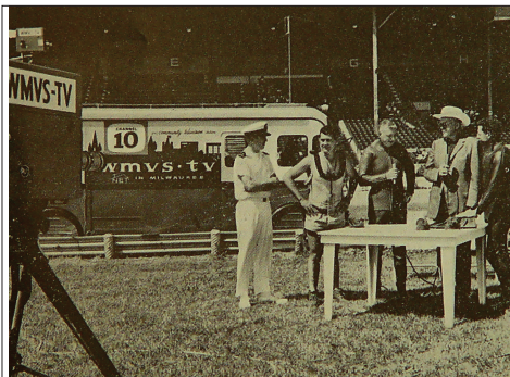
Figure 7.1 Up until the 1970s the only practical way of getting a television camera into the field, and supporting it once it got to its location, was to install it in a truck. We have already elaborated on the fact that cameras used to come as three fairly heavy pieces of equipment: the camera head (the part of the camera visible in this photo), a camera control unit and a power supply. In addition it took one other piece of equipment to make the camera work, a "sync" generator. Until the late '60s, high-end cameras couldn't create images by themselves without a half dozen "drive" signals from that generator.
